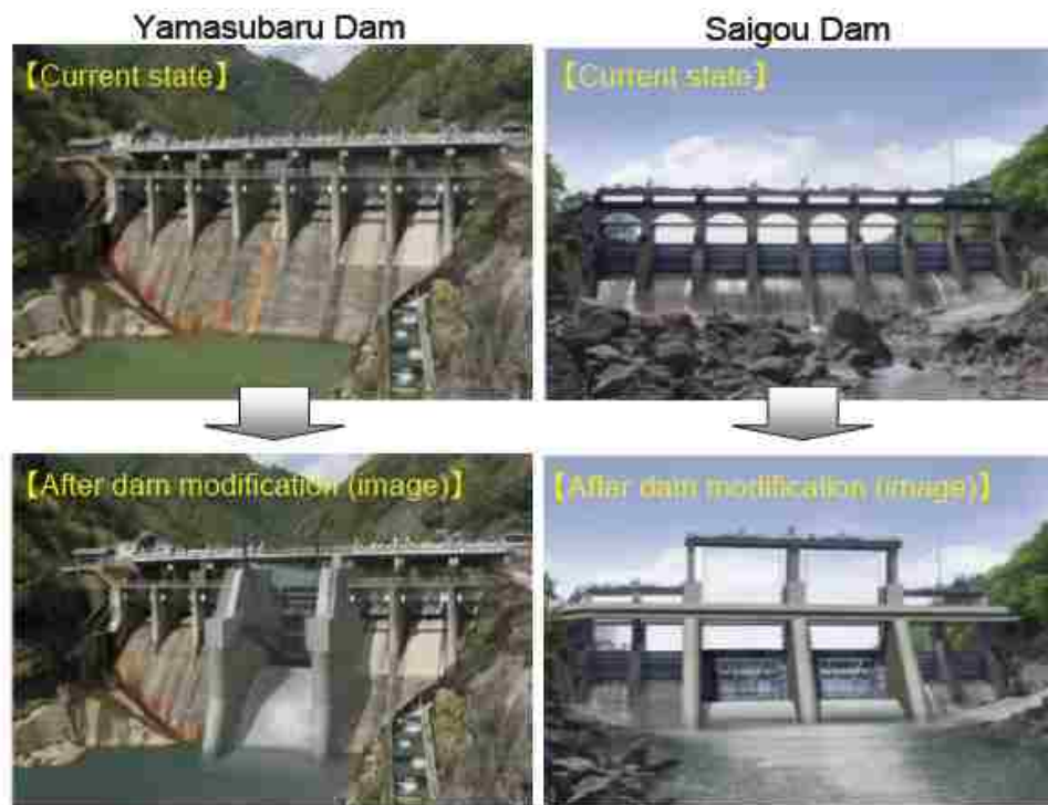
Figure 3-6: Dam retrofitting for Yamasubaru and Saigou Dams (Sumi et al. 2015)
